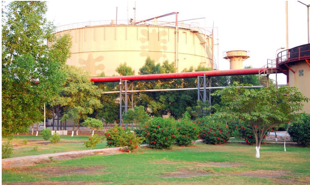
Effluent Treatment Plant
